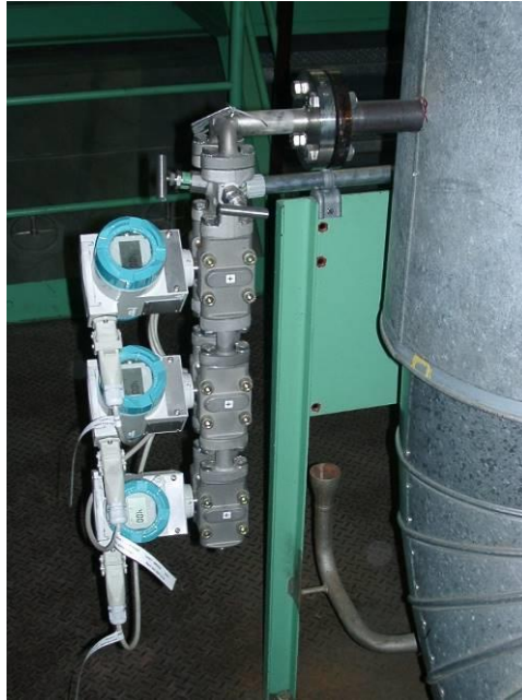
Differential pressure measurement with 3-fold splitting range
