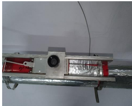
Figure 16: Gluing the free area inside the mounting rail.
